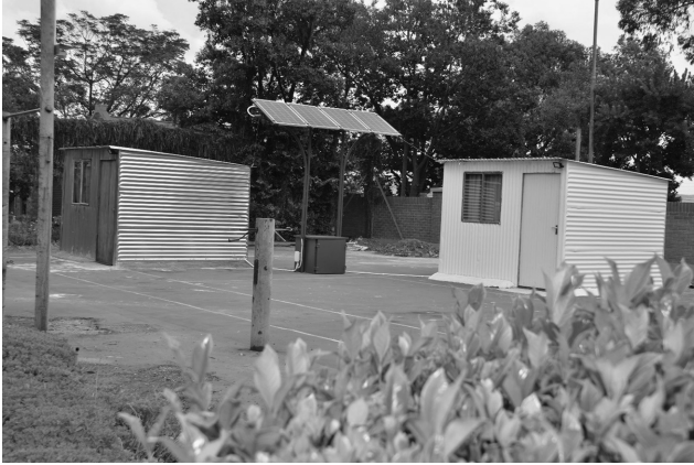
Figure 1.1 Unisa demonstration site for three clean-energy solutions for households: solar, biogas and cool coatings. (Source: Kimemia, 2019.)
